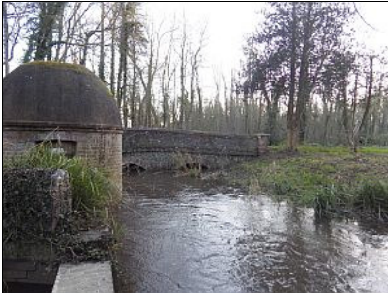
The River Glaven at Bayfield Bridge. The building on the left houses a Victorian hydraulic ram machine which once supplied Bayfield Hall.
