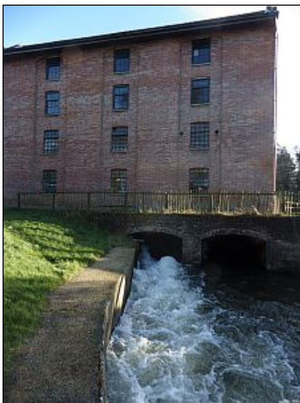
Letheringsett Mill, showing two mill races. The one on the right houses the water wheel, the one on the left is a bypass used when the wheel is not in operation.
