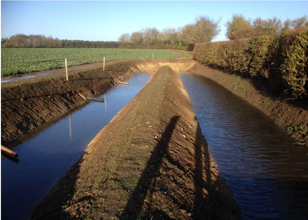
ROADSIDE SEDIMENT TRAP, SALLE PARK ESTATE, NORFOLK
