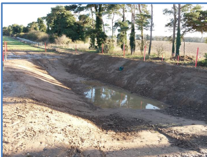
Figure 4. Silt trap (1) installed in December 2017.
