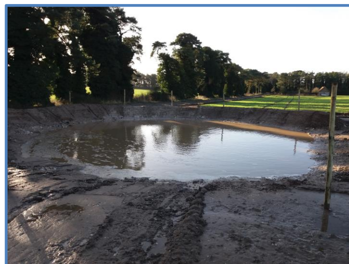
Figure 5. Silt trap (2) installed in December 2017, complete and capturing run off.
