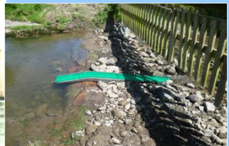
© Environment Agency. An example of an eel pass
