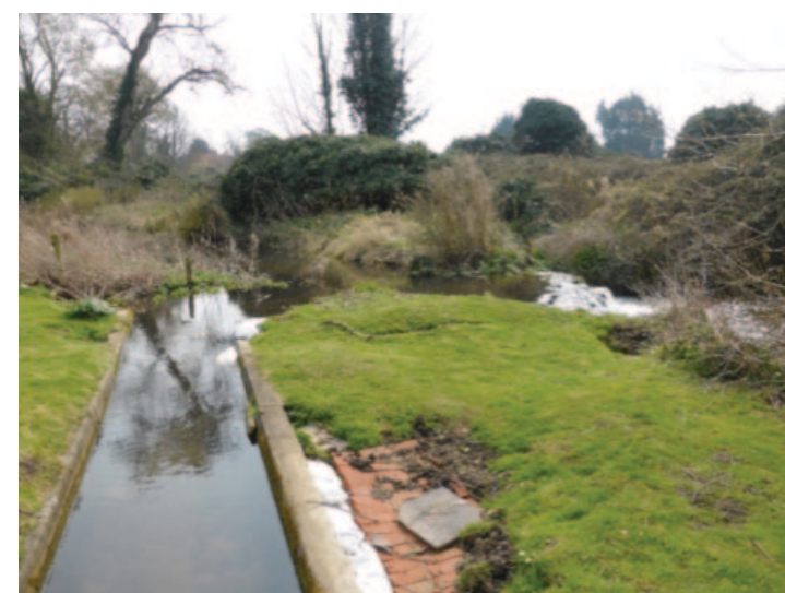
Impoundment near Pocahontas Lake, Heacham. Channel flowing towards photo flows through the fishing lake and then back into the river. The impoundment will prevent course fish passage, and would be a barrier to migratory species under most flow conditions
