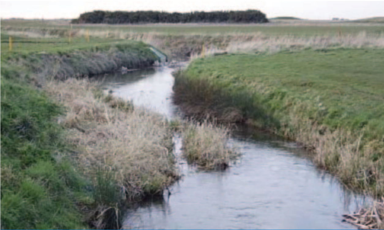
The river is channelled where it passes through Heacham golf course, and has lost natural connection with its floodplain.
