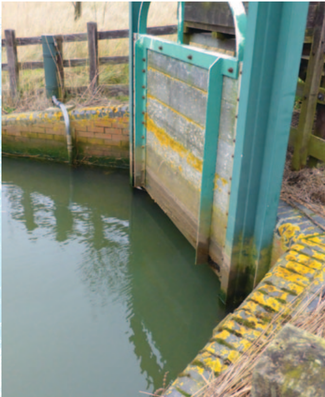
Photo 23. Tidal sluice at Hun outfall.
