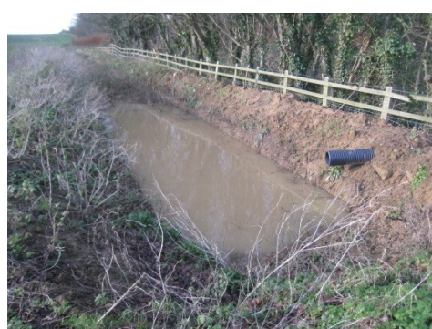
(Left) Map showing the run-off in an arable fields and where silt traps were constructed. (Middle) One of the silt traps constructed in the mapped field. (Right) Silt trap collecting run-off off a long farm track.
