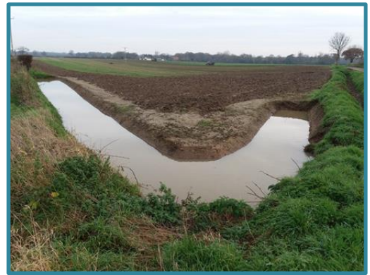
Figure 5. Field corner bund after rainfall, Fleggburgh
