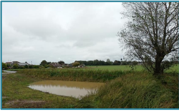
Figure 3. Bund after construction and following heavy rain in October 2020 © Neil Punchard
