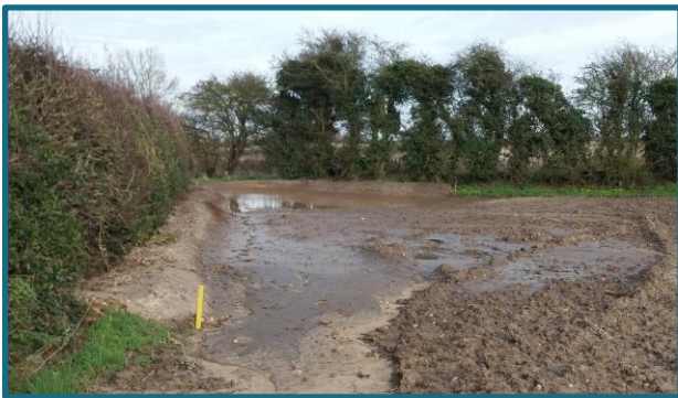
Figure 4. Field corner bund, West Somerton
