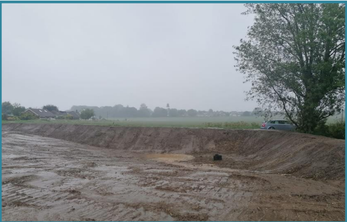
Figure 2. Bund during construction in June 2020 © Neil Punchard
