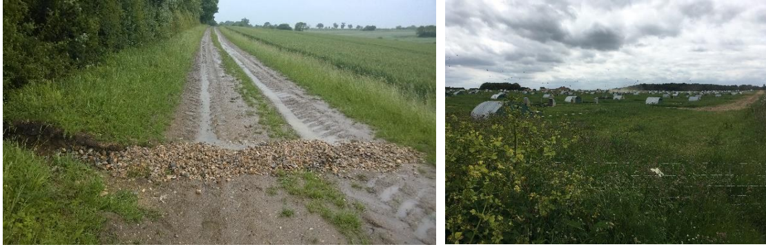
Cross drains in track to divert surface flow (left). Wide green margins for intercepting runoff (right).
