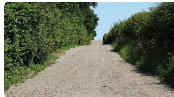
Figure 2b. Farm track after works
