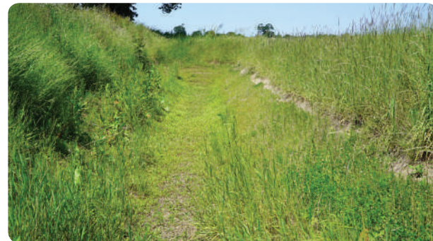
Figure 3. Silt trap at bottom of track (following drought conditions)
