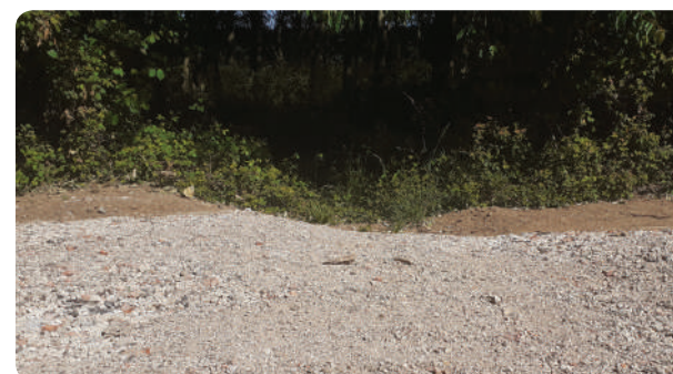
Figure 2c. Track cross drain into adjacent wooded area
